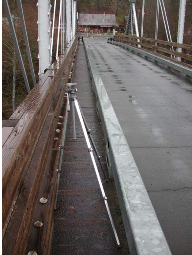
Figure 3.1. Old Lewiston Bridge photopoint #1100OLB1 observation point monument.
