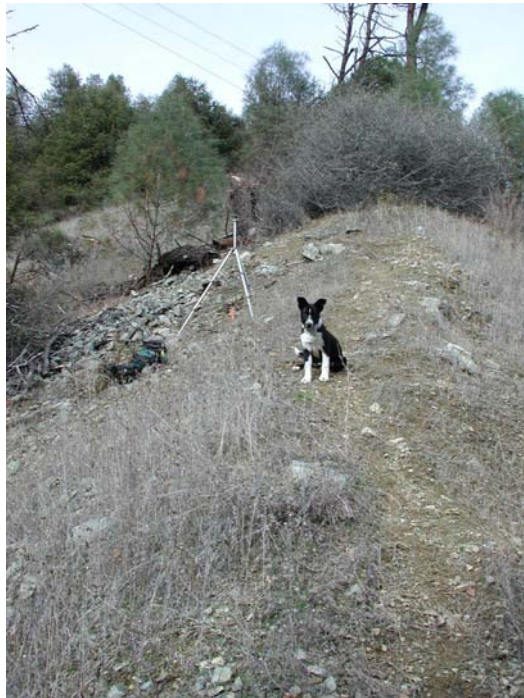
Figure 1.2. Lewiston Dam photopoint #1120LD1 and #1120LD2 observation point monument.
