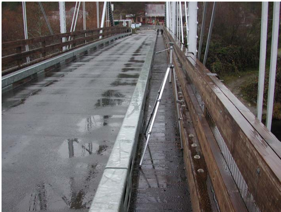
Figure 3.2. Old Lewiston Bridge photopoint #1100OLB2 observation point monument.
