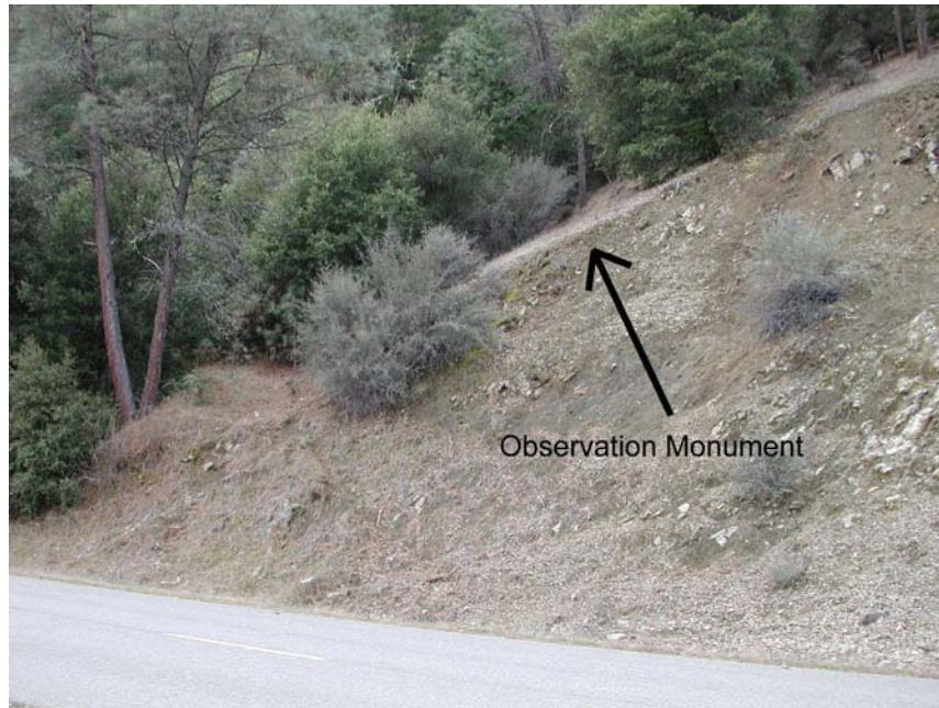
Figure 1.3. Lewiston Dam photopoint #1120LD3 observation point monument.
