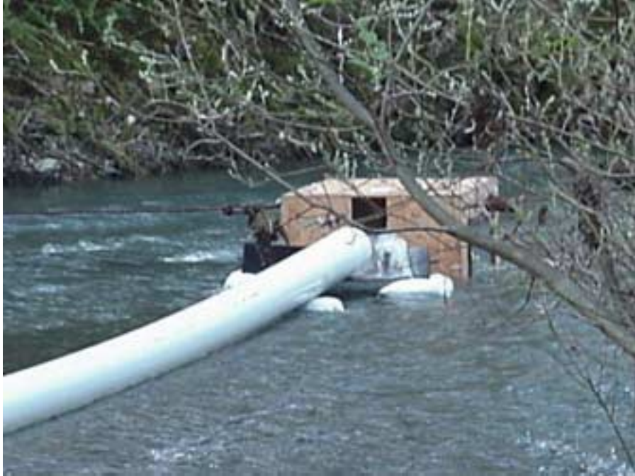
Figure 2. Water leaving PVC pipe and entering live box.
