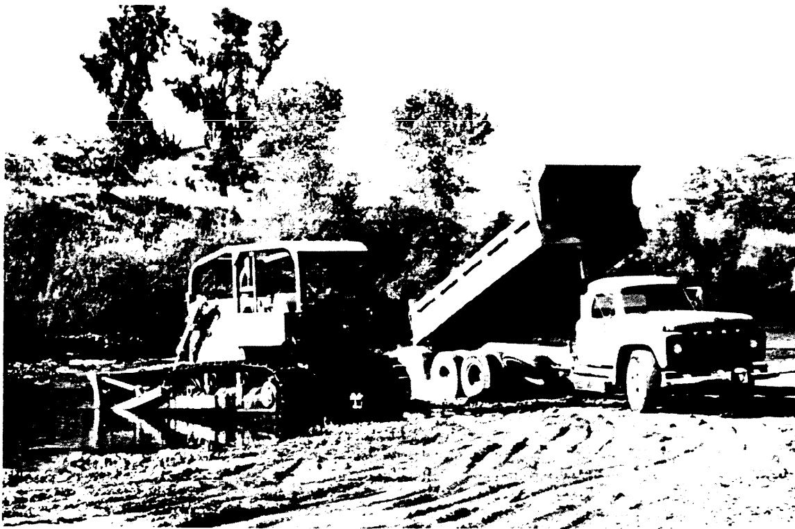
Spawning gravel rejuvenation project on the Feather River
