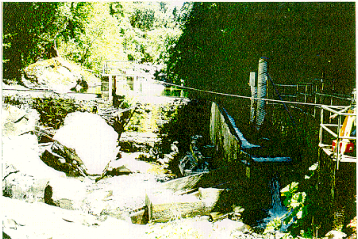
Photograph 2: Another view looking northeast at the downstream face of Eagle Canyon Dam. Note large basalt rocks in the stream channel; some are incorporated into the foundation of the dam.
